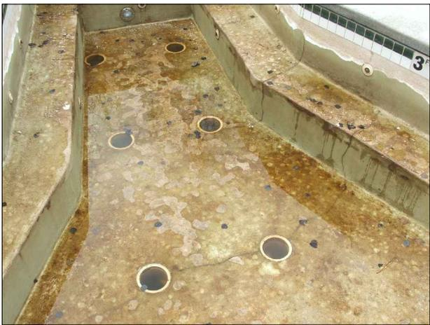
*Severe failure of plaster and algae staining as a result of not maintaining water balance over the winter.*
